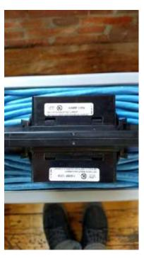
Center legs are cut out in the middle to allow cables to pass through to the next tray
