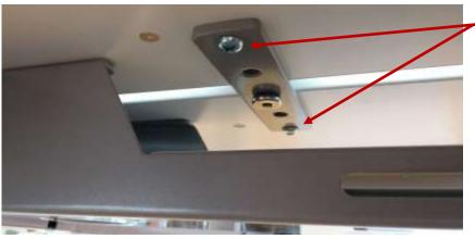
Install two wood screws on each end of 5 hole bar to bottom side of worksurface
